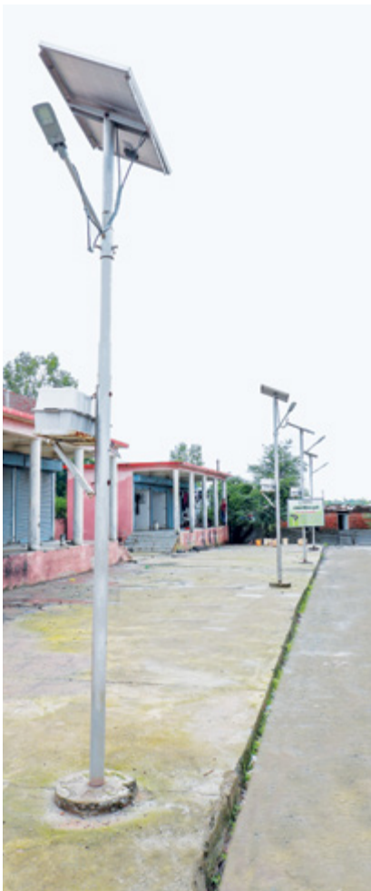
Solar Lights installed in Budhni (MP) region
